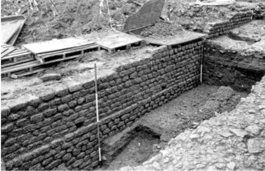
Above: View from Walcot Street of the Aldridge's building under refurbishment, and in the foreground the Roman walling running towards the river. The graves were found in the deeper
